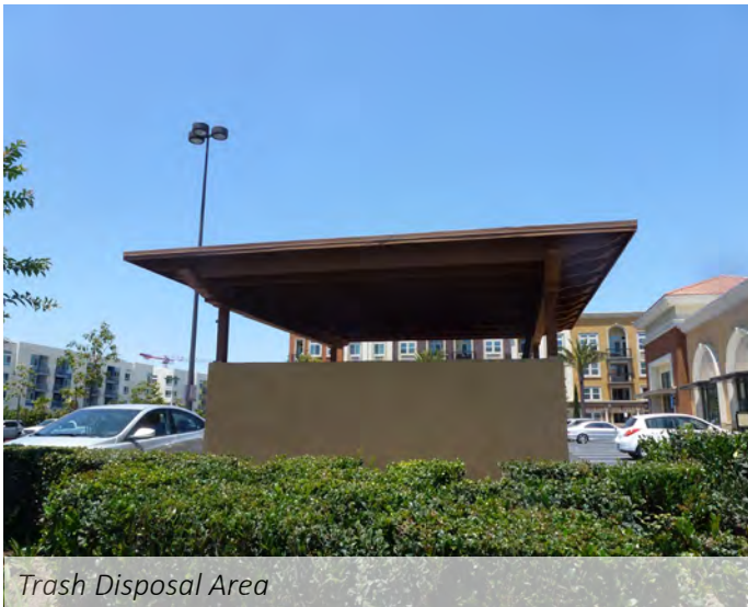
Trash Disposal Area
