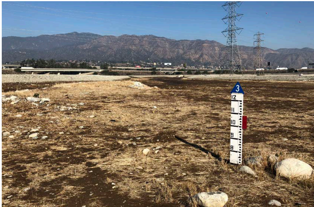
Basin 3E at Santa Fe Spreading Grounds
