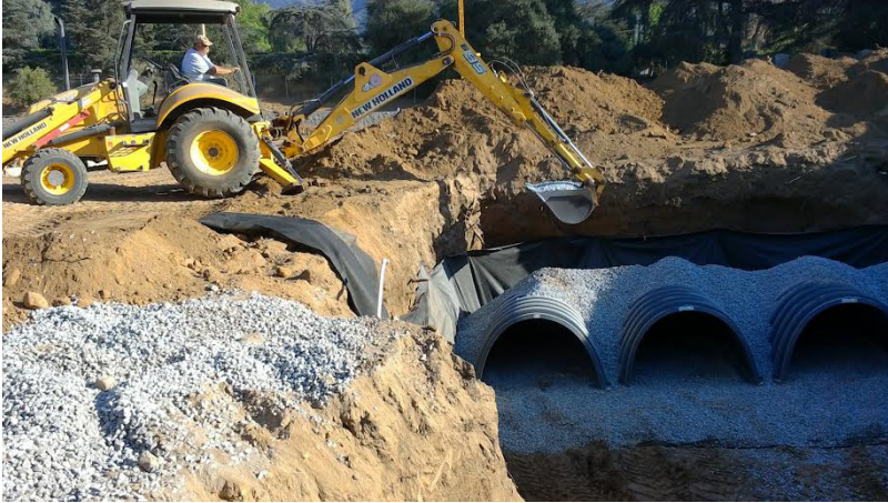
Stormwater Infiltration in City of Bradbury
