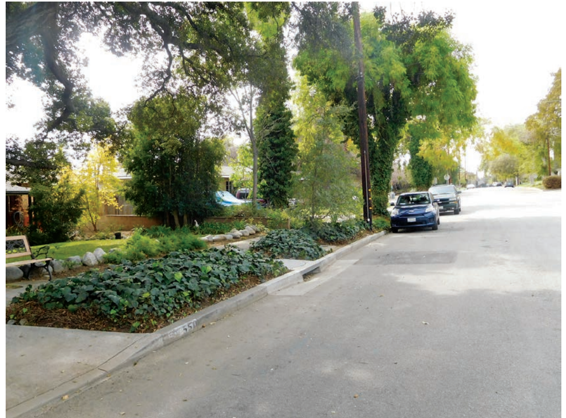
Dry Well Treating Road Runoff and Recharging Groundwater in Sierra Madre
